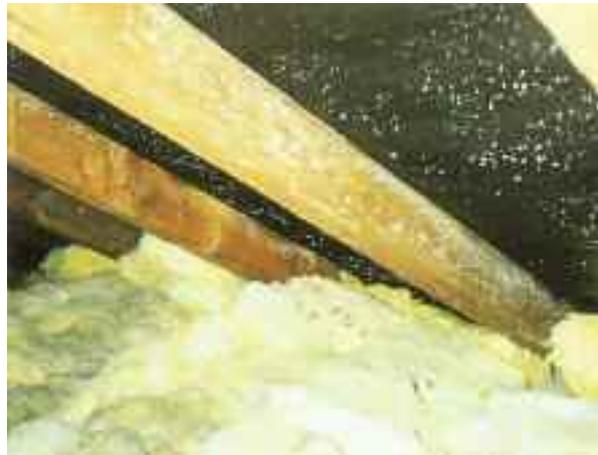
Reduced ventilation in this case caused by blocked eaves ventilation gaps can give rise to condensation and mould growth.
