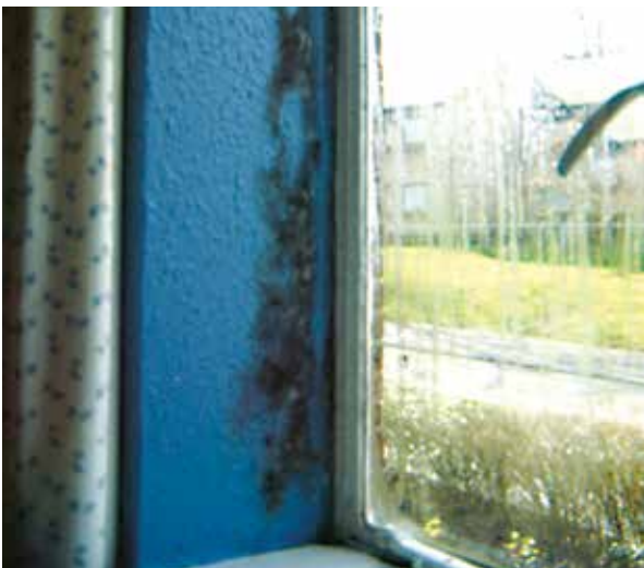
Unightly Mould Growth as a Result of Thermal Bridging.
